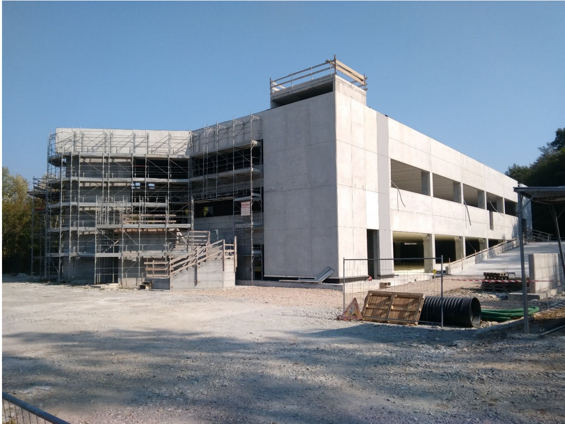
Fig. 1 –Overview of the building during advanced construction stage
