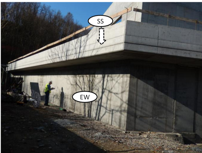
Fig. 2 – View of external wall and suspended slab (behind parapet)
